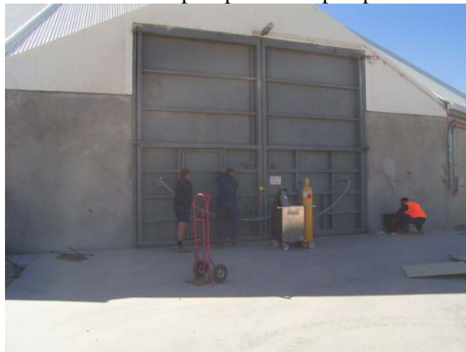
Figure 3: (from L to R) Steve Hussey (SunRice), Darren Poole (SunRice) and William Shore (GasApps) sealing door and setting up phosphine introduction equipment
